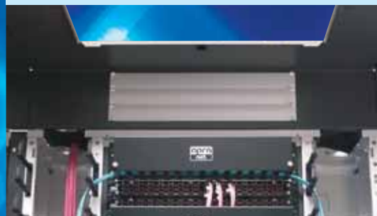
Internal view cooling corridor
